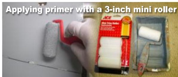
Mini rollers leave the surface smoother than a brushed surface, but not as smooth as a sprayed surface. Mini rollers are excellent for applying primer because the primer
