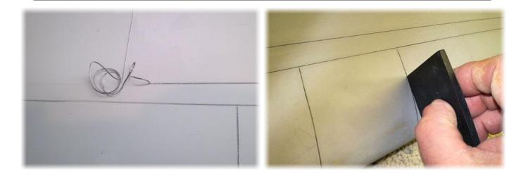
For overlapped panels, apply one or more layers of regular masking tape and apply primer over one edge of the tape. When dry, remove the masking tape and lightly sand the edge.
